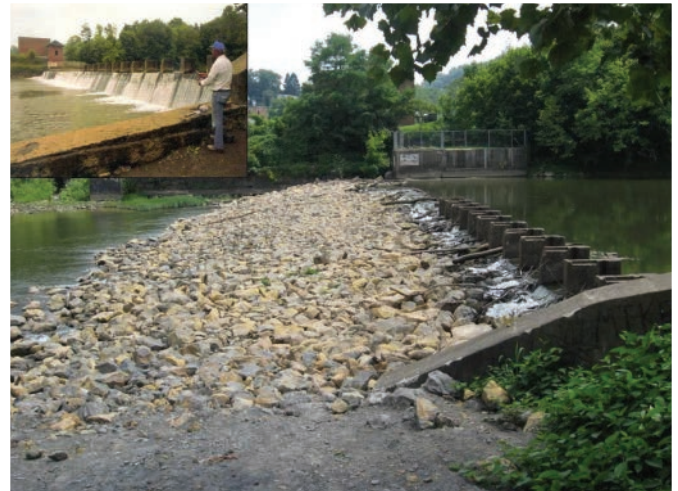
Low head run-of-the-river dam on the West Fork River, Harrison County, W.Va.
