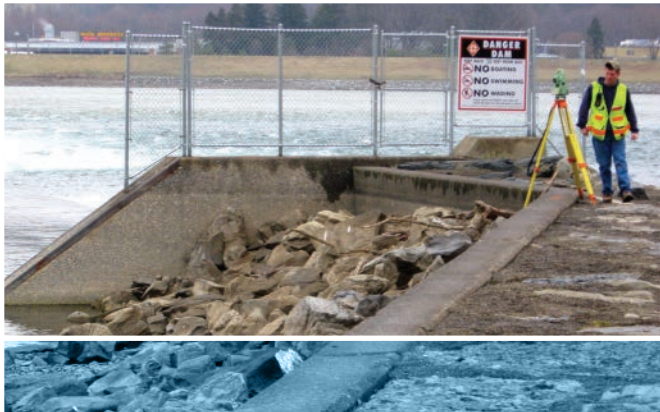
Moveable crest inflatable dam, Sunbury, Pa.
