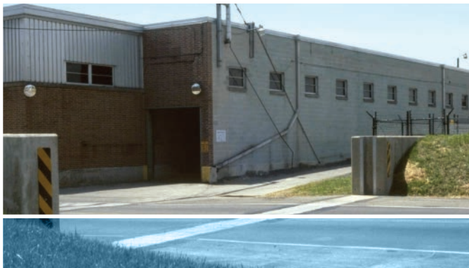
Stoplog closure structure, Corderus Creek, York, Pa.
